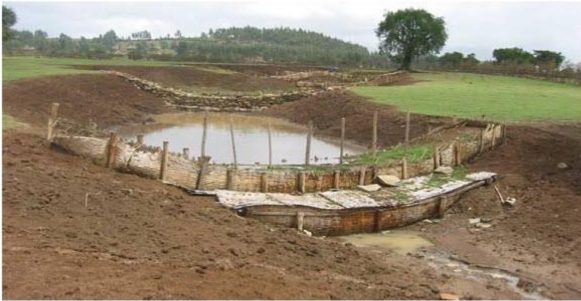
Fig. 1.3. Brushwood check dam.
