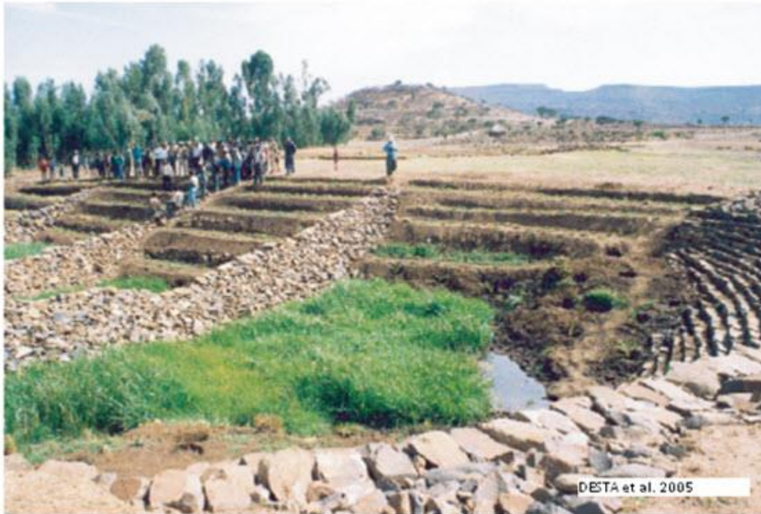
Fig. 1.1. Gully reshaping and filling. (Source: https://energypedia.info/images/a/aa/GullyReshapingRevegetation.png )
