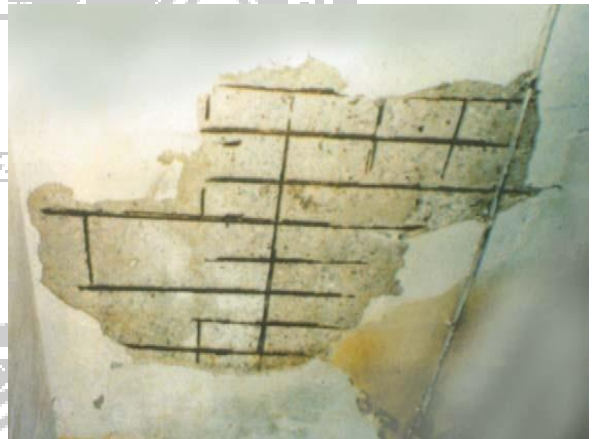
Example of delamination of concrete cover
