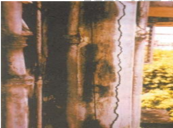
Rusting of reinforcements
