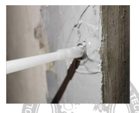
**Install injection ports:** Surface Ports (short rigid-plastic tubes with a flat base) serve as handy entryways for getting the repair material into the crack.
