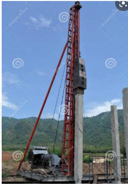
Figure-1: Pile driving using hammer
