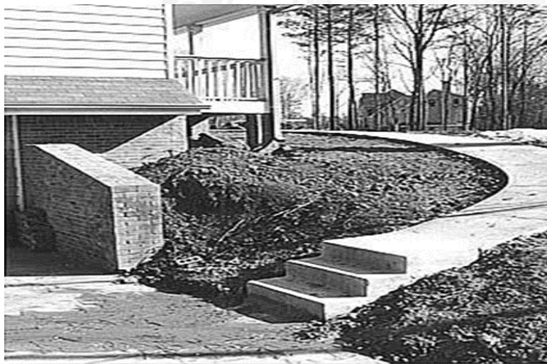
Retaining wall, steps, and walk.
