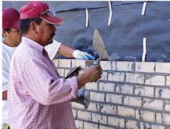
Applying a brick veneer to wood frame construction.
