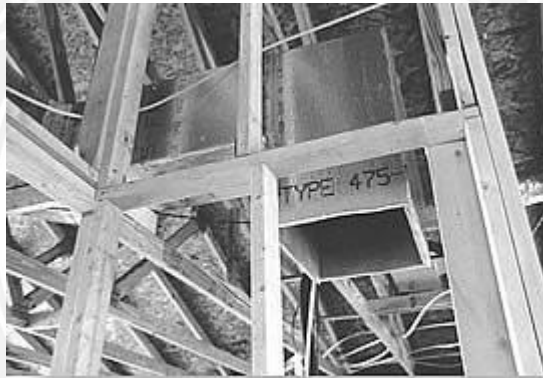
This is an insulated duct board that can be cut with a knife, which makes installation easier.
