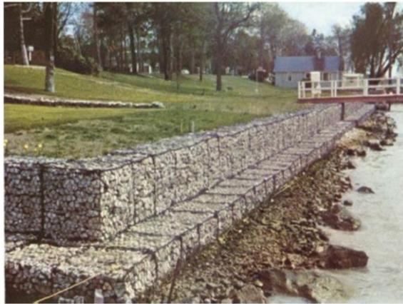
Bulkhead structure constructed by Gabion mesh boxes
